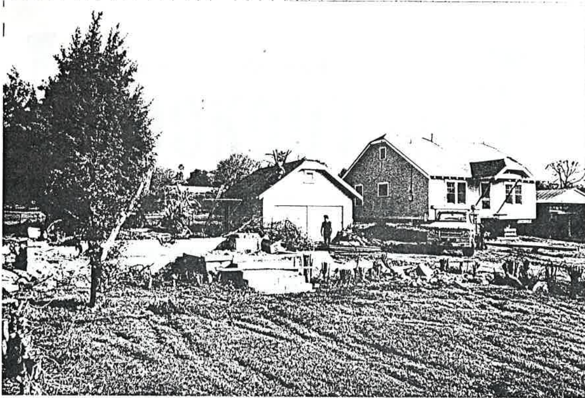
Original foundation, garage, and new location.
