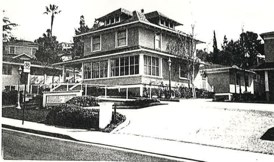
The restoration which began in 1985 included the removal of the attached garage.
