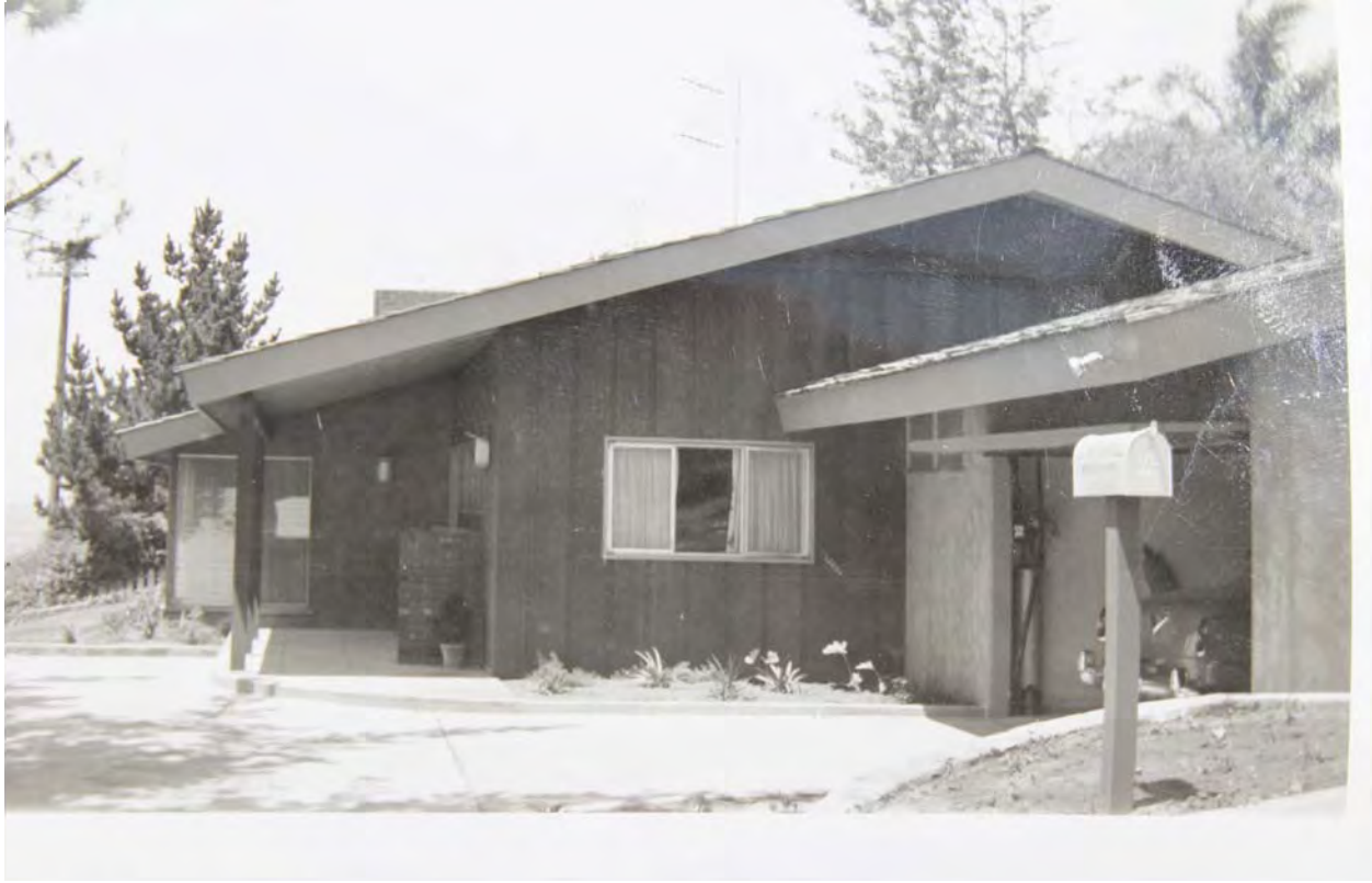
Fig.47: Finished house looking north. Note original lights in entry.
