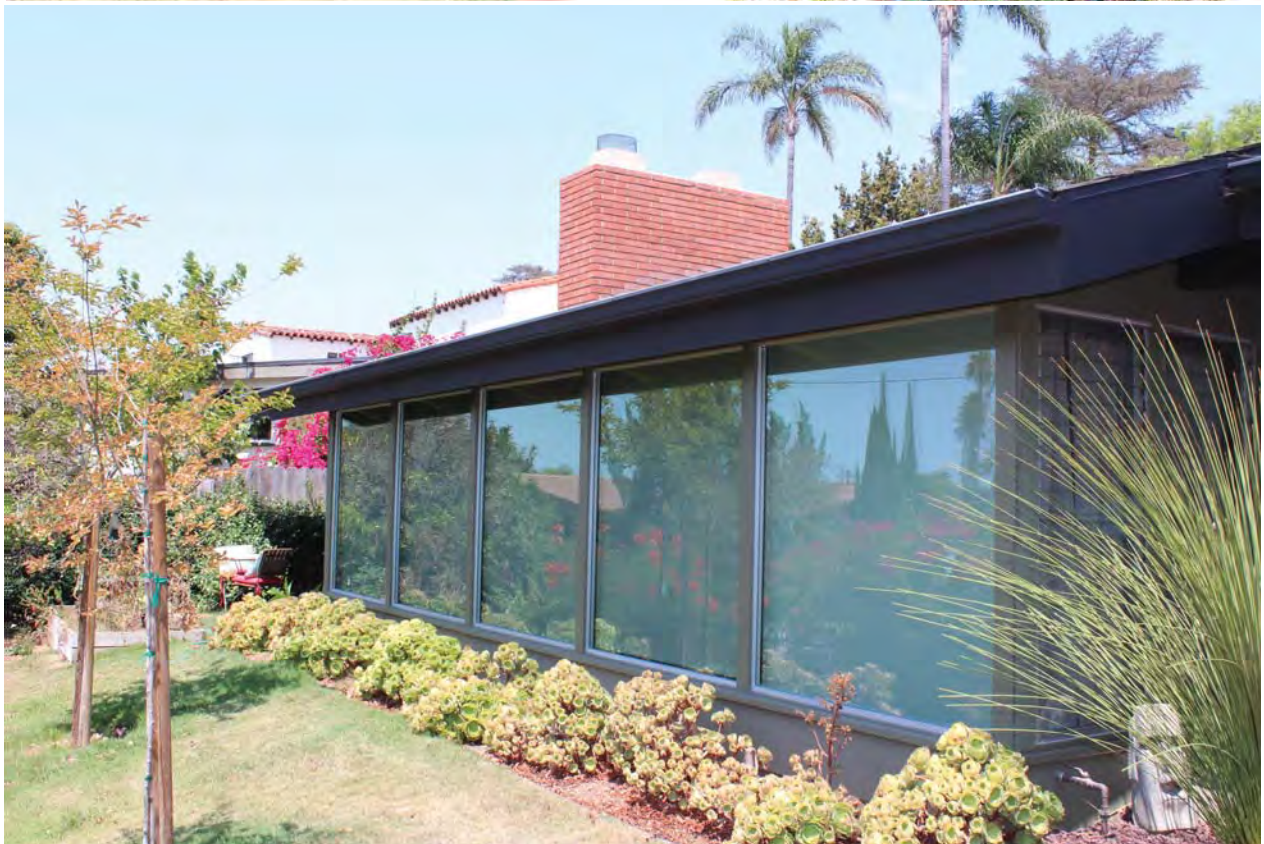
Fig. 6: Livingroom windows looking northeast.
