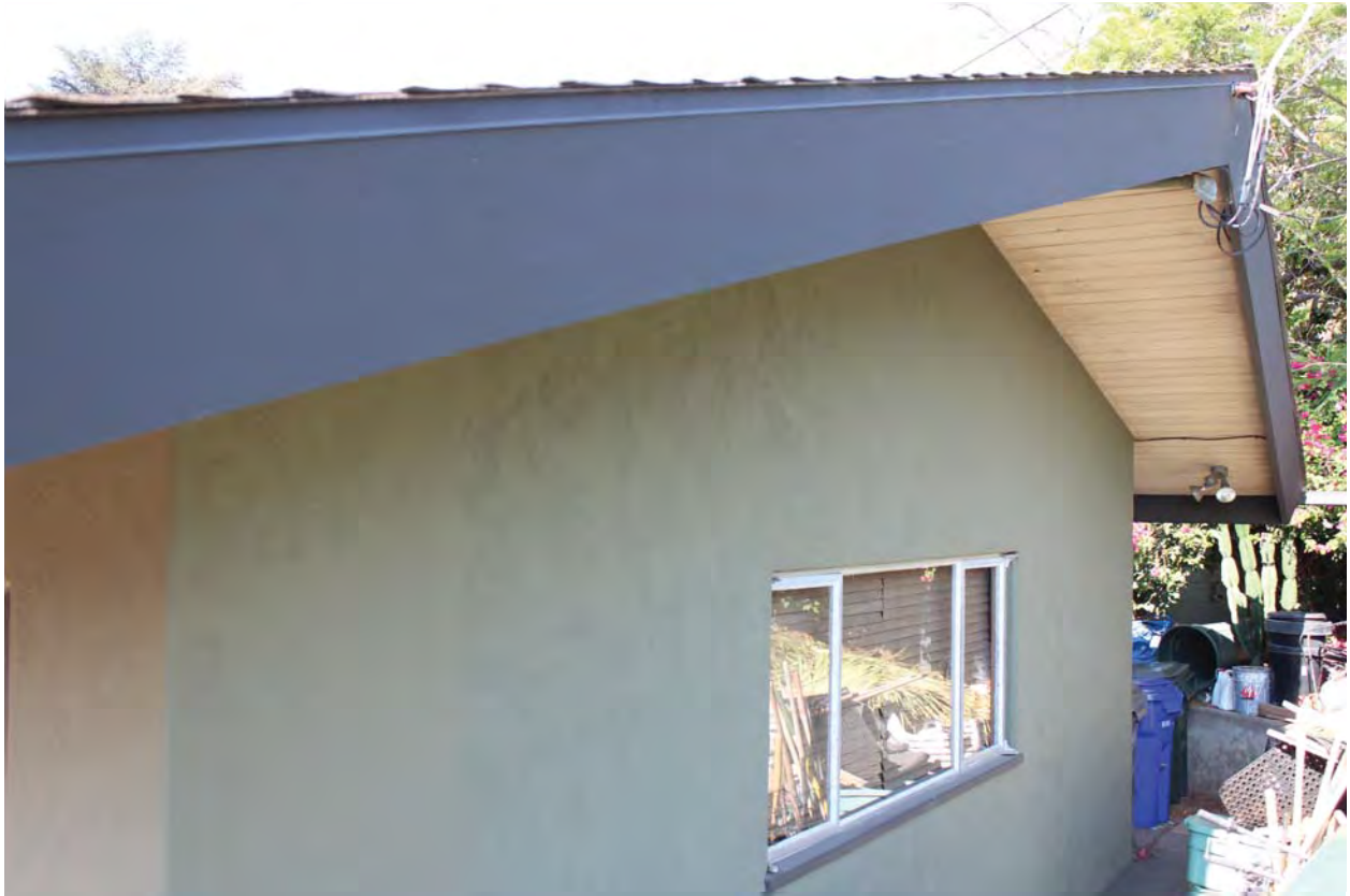
Fig. 16: South side of garage looking east.
