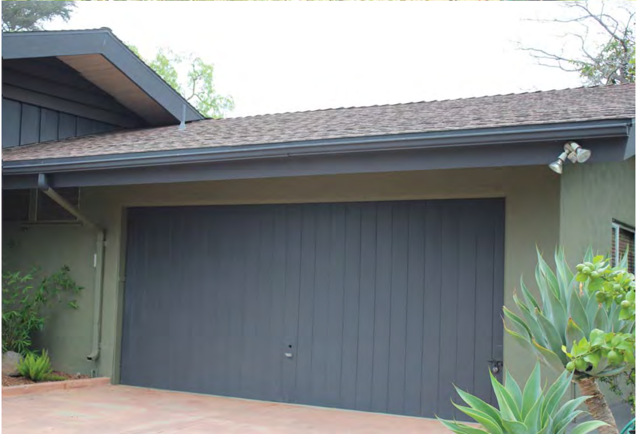
Fig. 8: Garage looking east.
