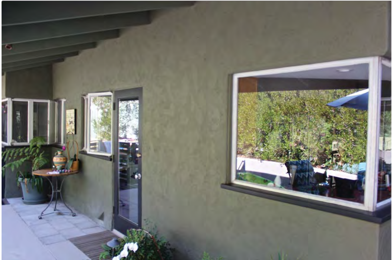
Fig.15: Back of house looking west.
