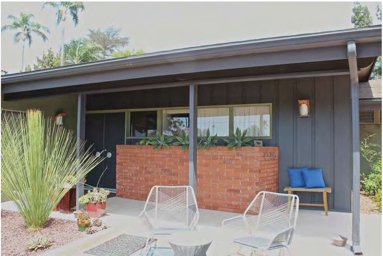
Fig. 4 View of entry looking east.
