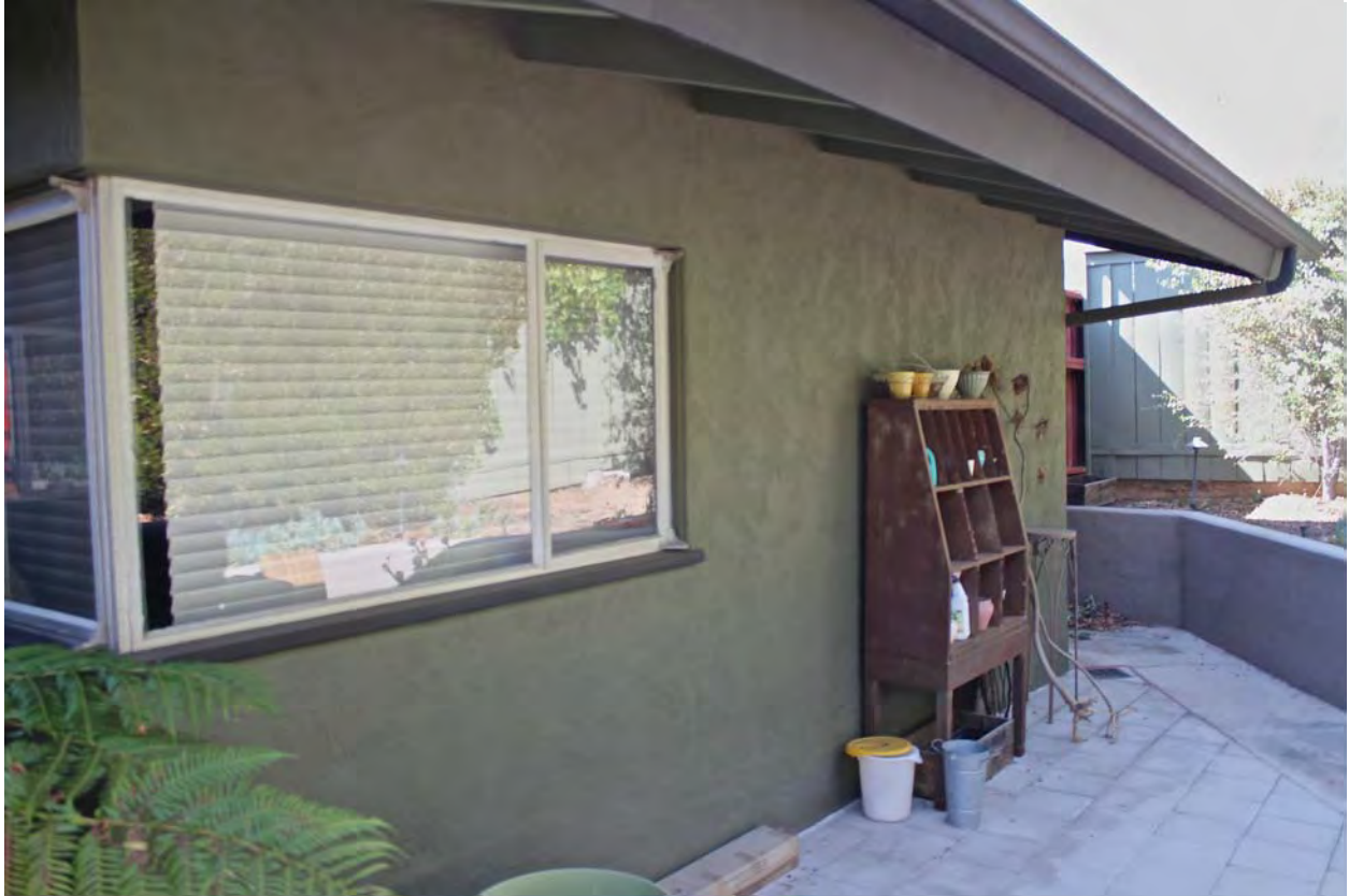
Fig. 11: Northeast corner of back of house looking northwest.
