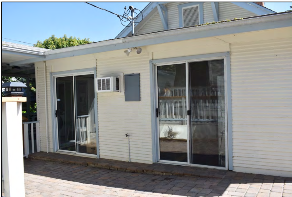
Photo 8: View east of the west elevation of the main dwelling showing enclosed porch and sliding glass doors. This volume is regarded as non-contributing.
