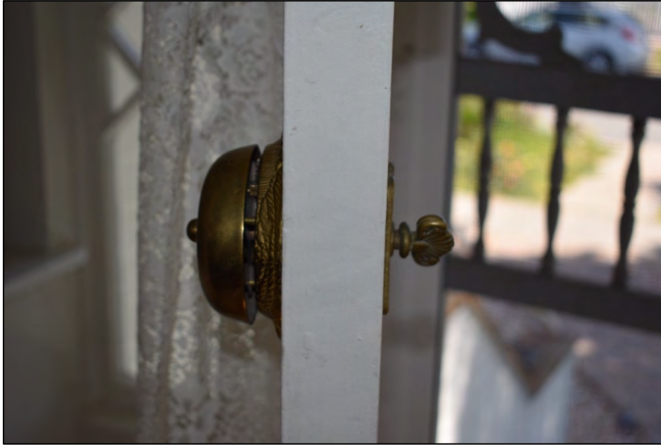
Photo 12: View of original doorbell hardware.
