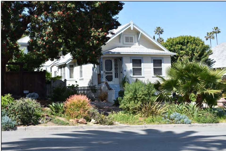
Photo 2: View northwest of the east and south elevations showing the enclosed front porch.
