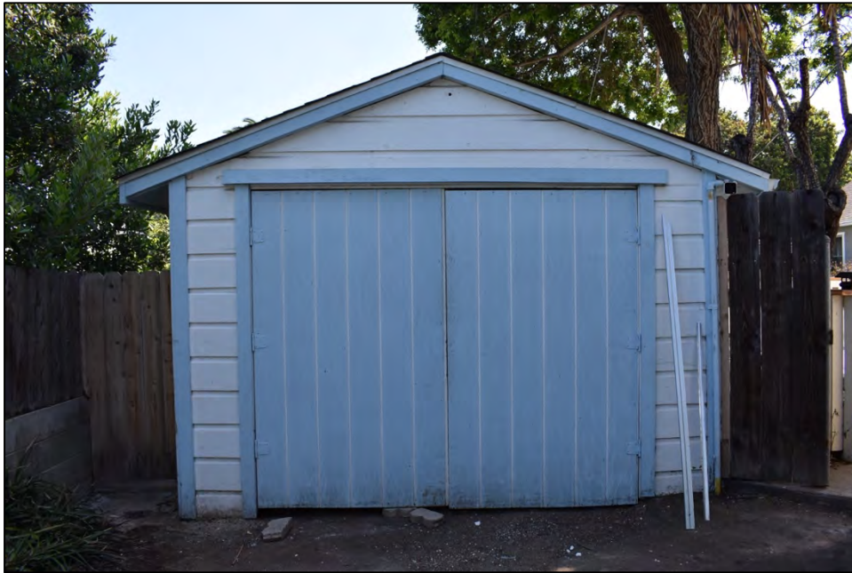
Photo 16: View east of west elevation of garage.
