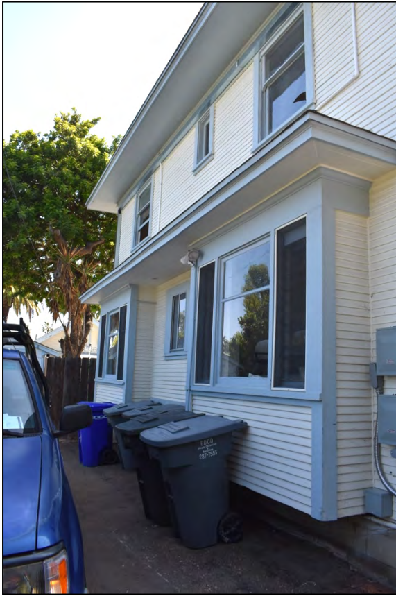
Photo 18: View east of the north elevation of the rear building showing bay windows with tripartite windows, shared hipped roof, and horizontal board siding.
