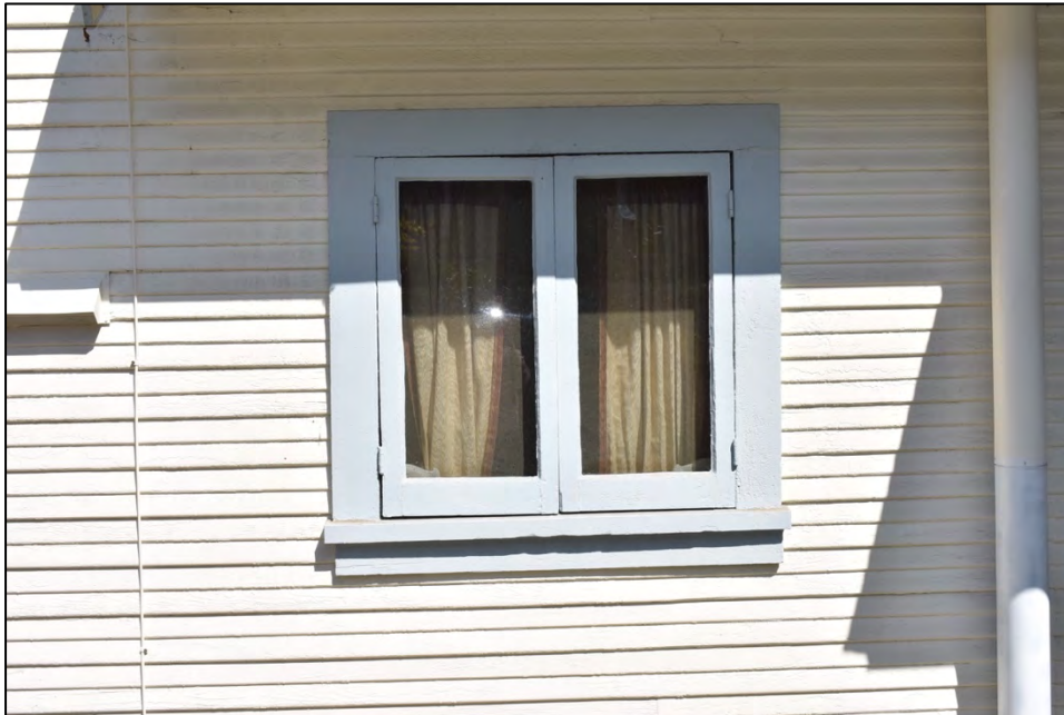
Photo 13: Example of original casement window with simple wood framing.
