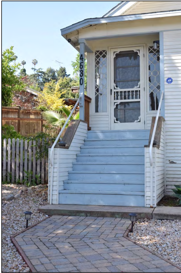
Photo 3: View of the front entrance with the restored front steps, wood railings, and pony wall.
