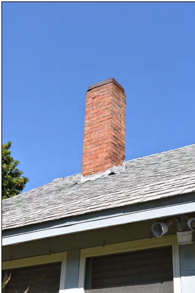
Photo 11: View of brick chimney.
