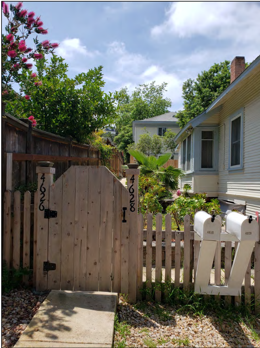
Photo 9: View northwest of south elevation showing bay addition and original wood sash window.
