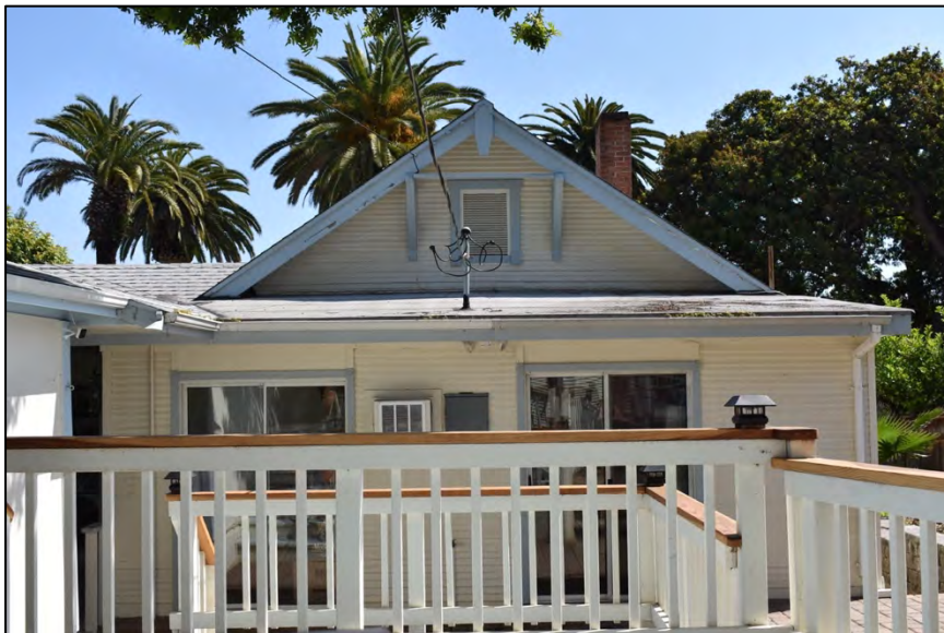
Photo 6: View east of west elevation of main dwelling.
