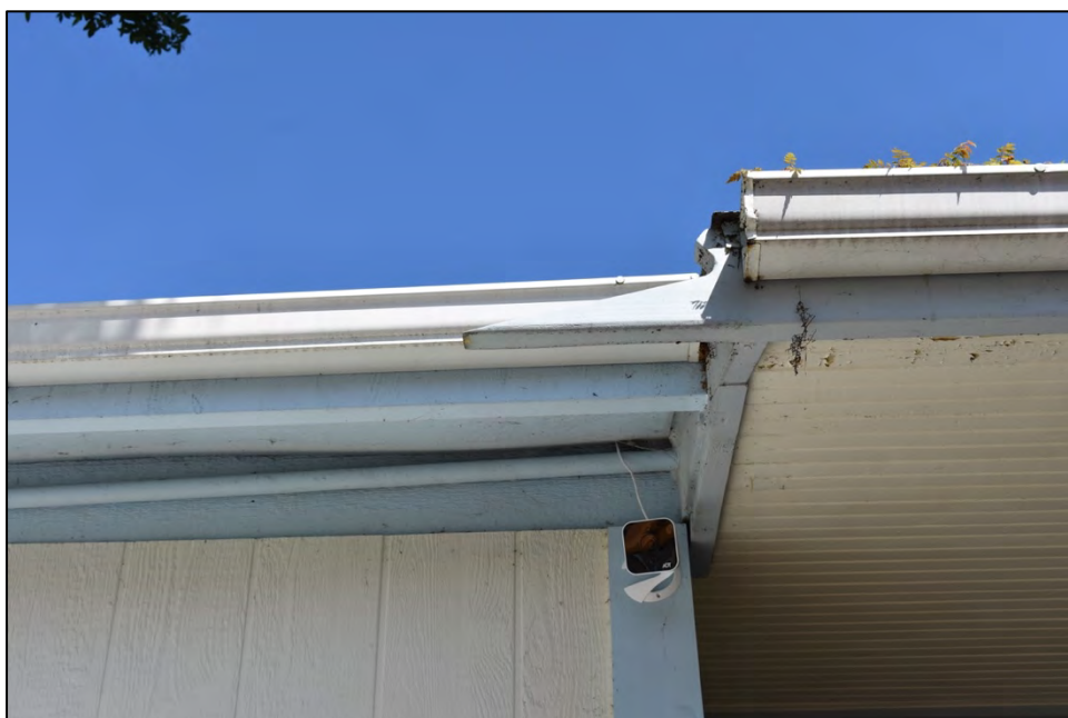
Photo 15: View of decorative fascia board. These points were removed from other sections of fascia boards.
