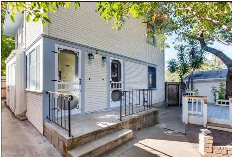
Photo 17: View west of the east and south elevations of 4626-2628 Date Avenue rear building.
