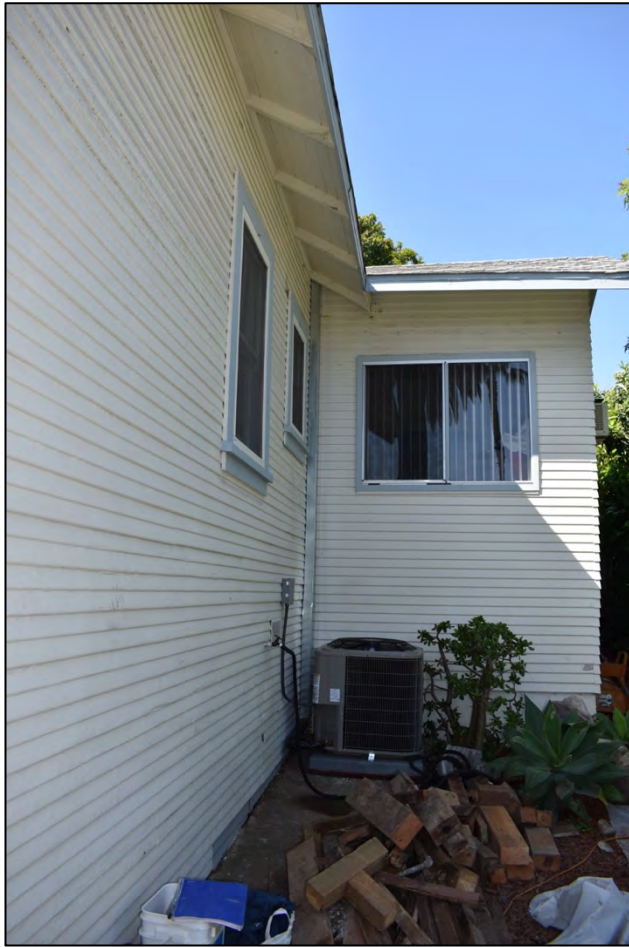
Photo 5: View west of north elevation showing bedroom addition and metal sliding sash window.
