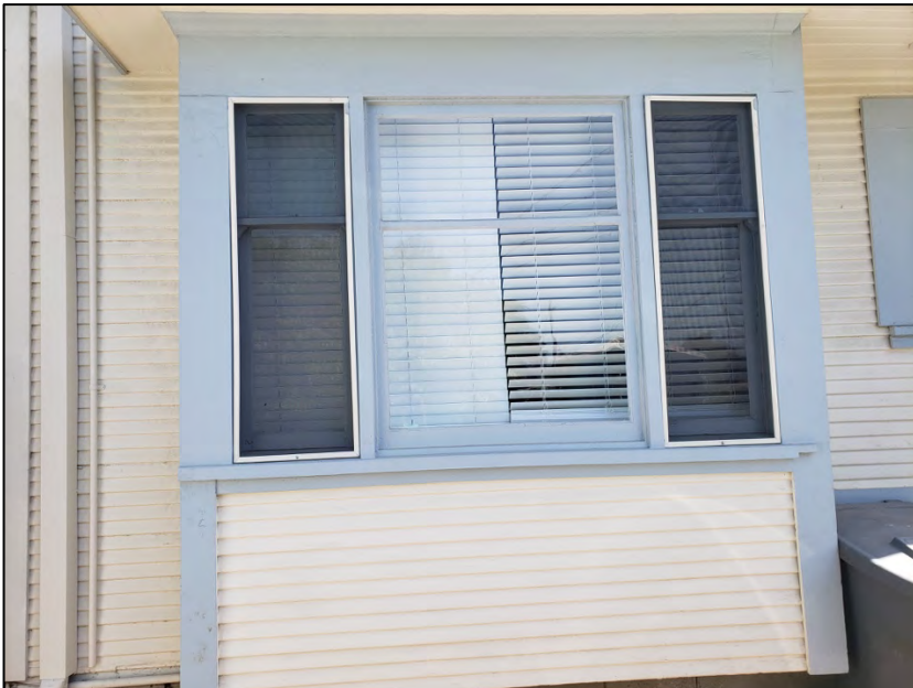
Photo 19: Close-up view of rectangular bay on the north elevation of the rear dwelling.
