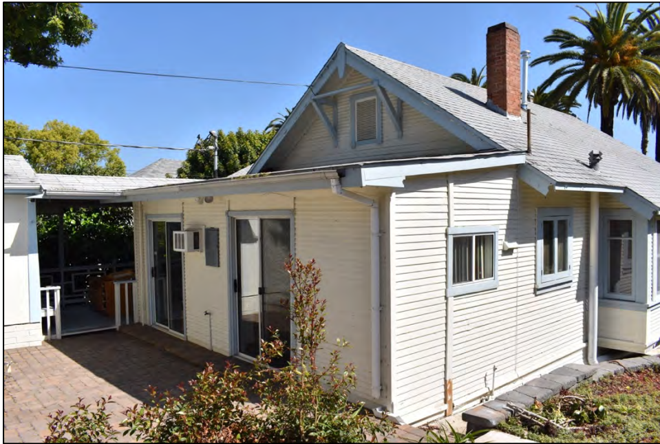
Photo 7: View northeast of west elevation showing non-contributing porch addition.
