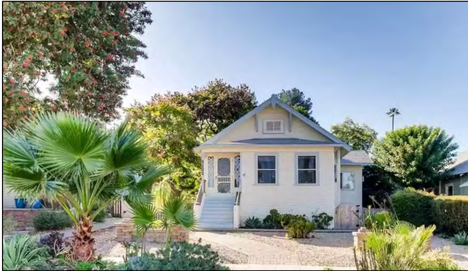
Photo 1: View west of east elevation from Date Avenue.
