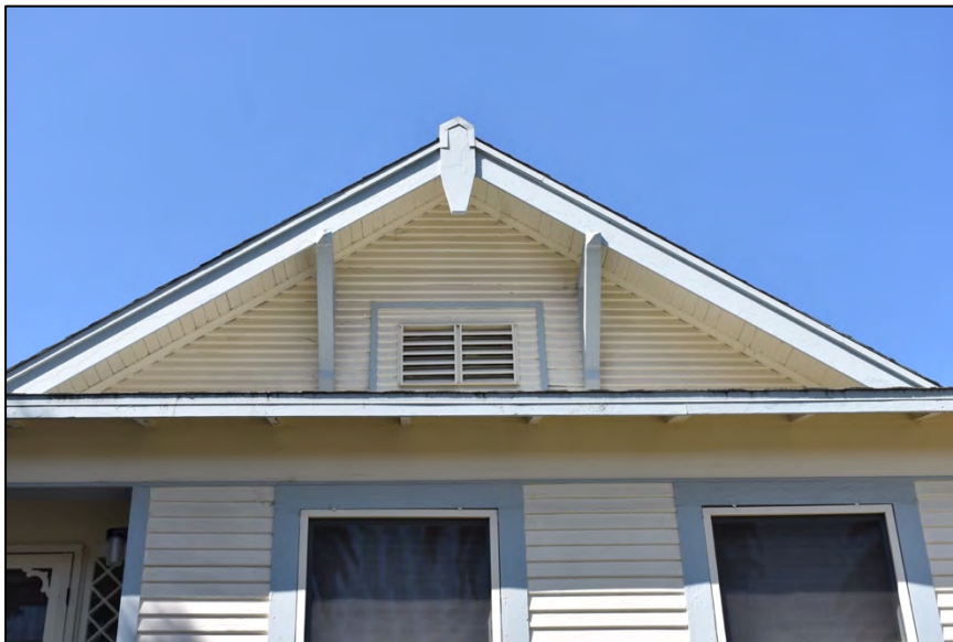
Photo 4: View of original knee brackets and louvered vent opening replacement of original fixed pane window.
