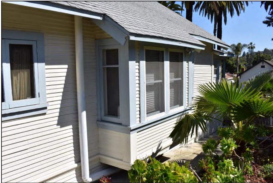
Photo 10: Close-up view of bay with casement and sash windows and horizontal board siding.
