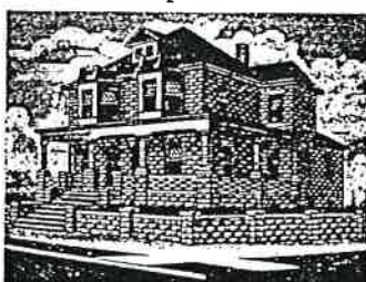
House, porch columns, balustrade and retaining wall all built of hollow concrete building blocks.
