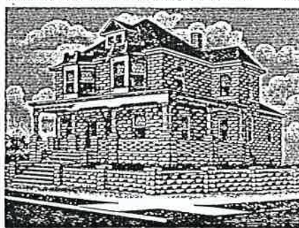
House, porch columns, balustrade and retaining wall all built of Mowbray Concrete Building Blocks.
