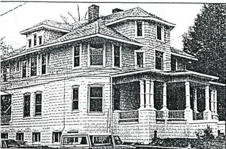
is quite popular for houses to be built with a concrete-block foundation porch, but a wood-frame upper storey finished with clapboards or shingles. A wood balustrade between piers is a variation on the all-concrete porch.
