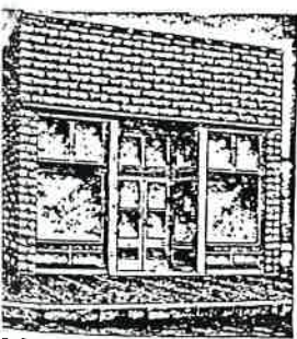
Building made of Concrete Building Blocks.
