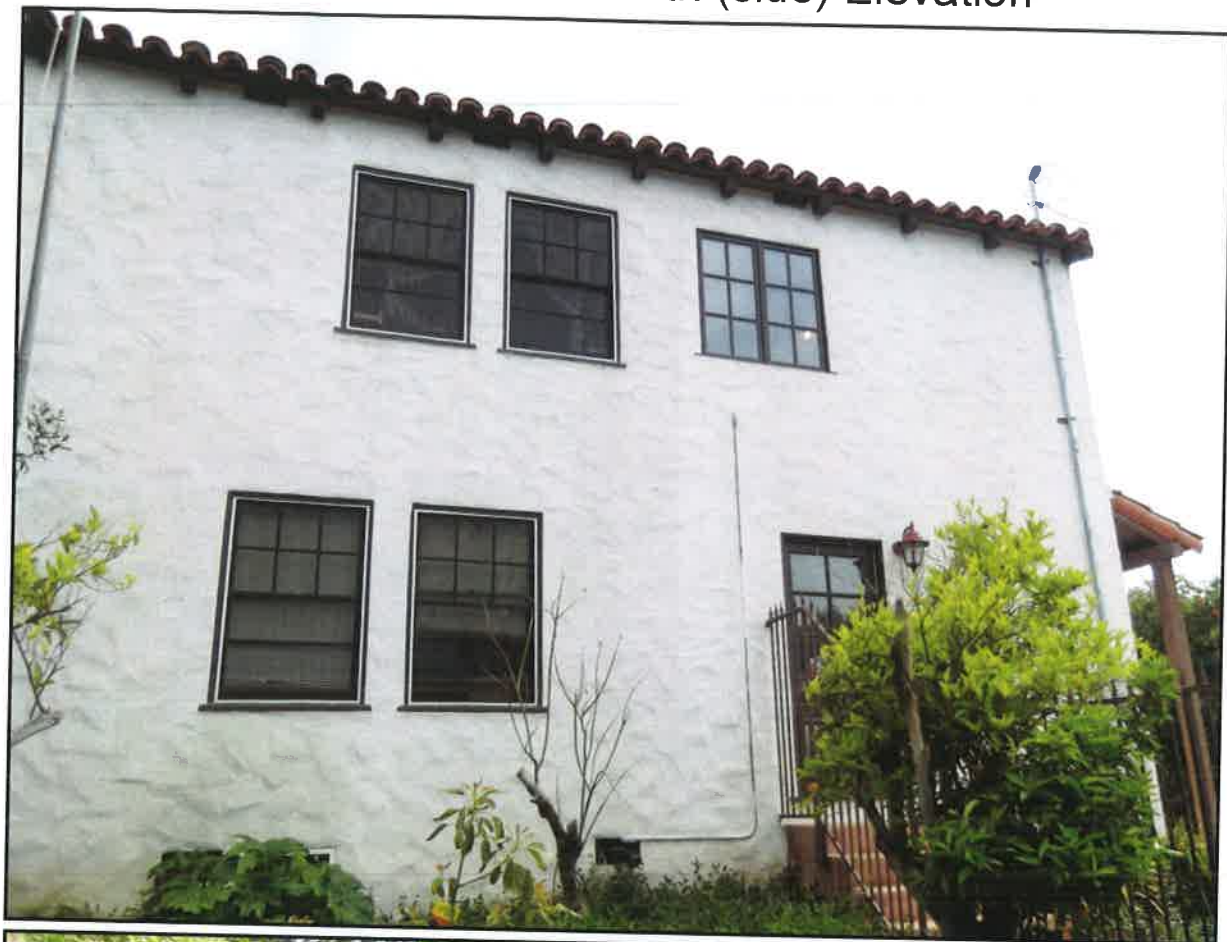
Current Photos - North (side) Elevation
