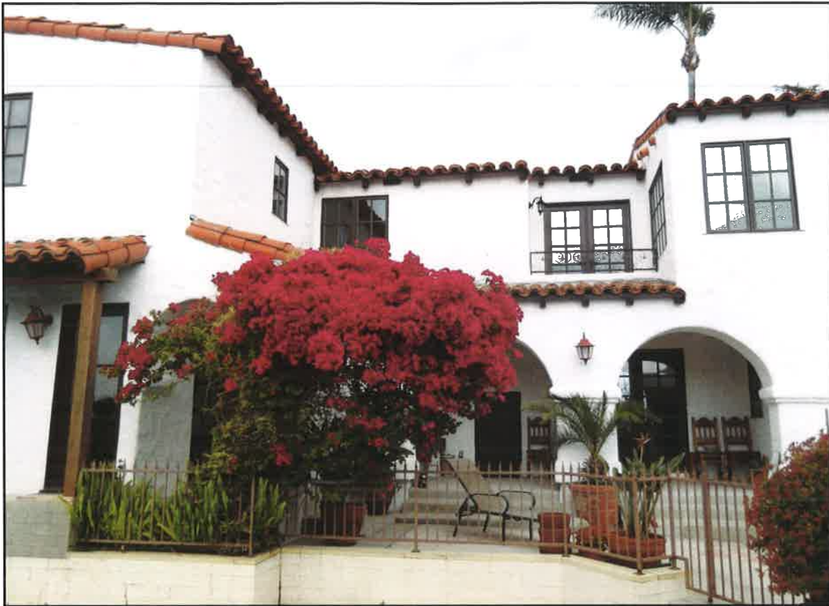
Current Photos - West (rear) Elevation
