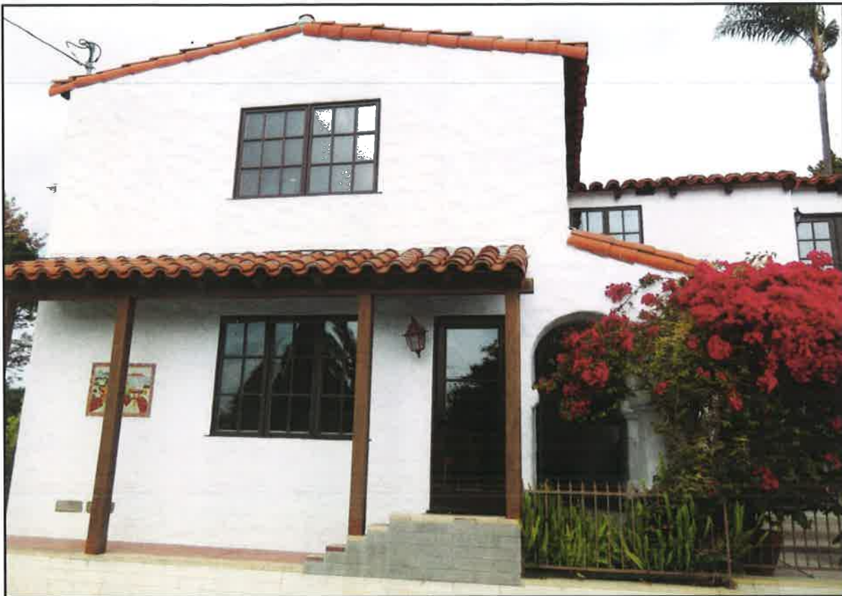
Current Photos - West (rear) Elevation
