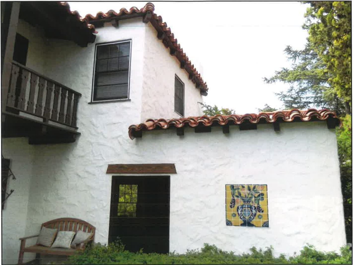
Current Photos - South (side) Elevation
