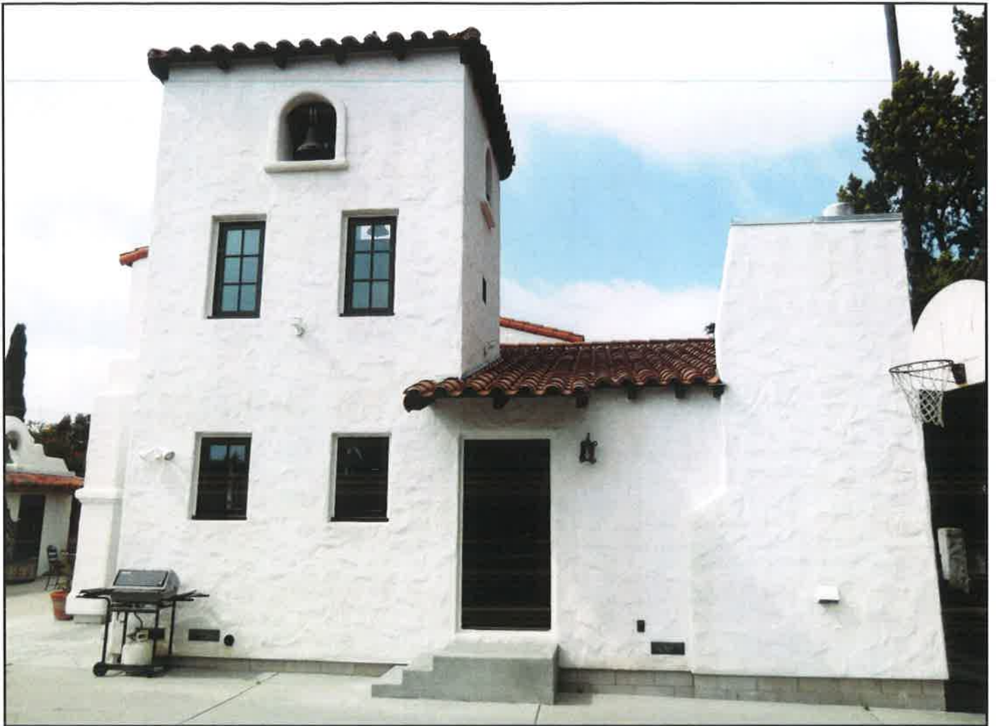
Current Photos - South (side) Elevation
