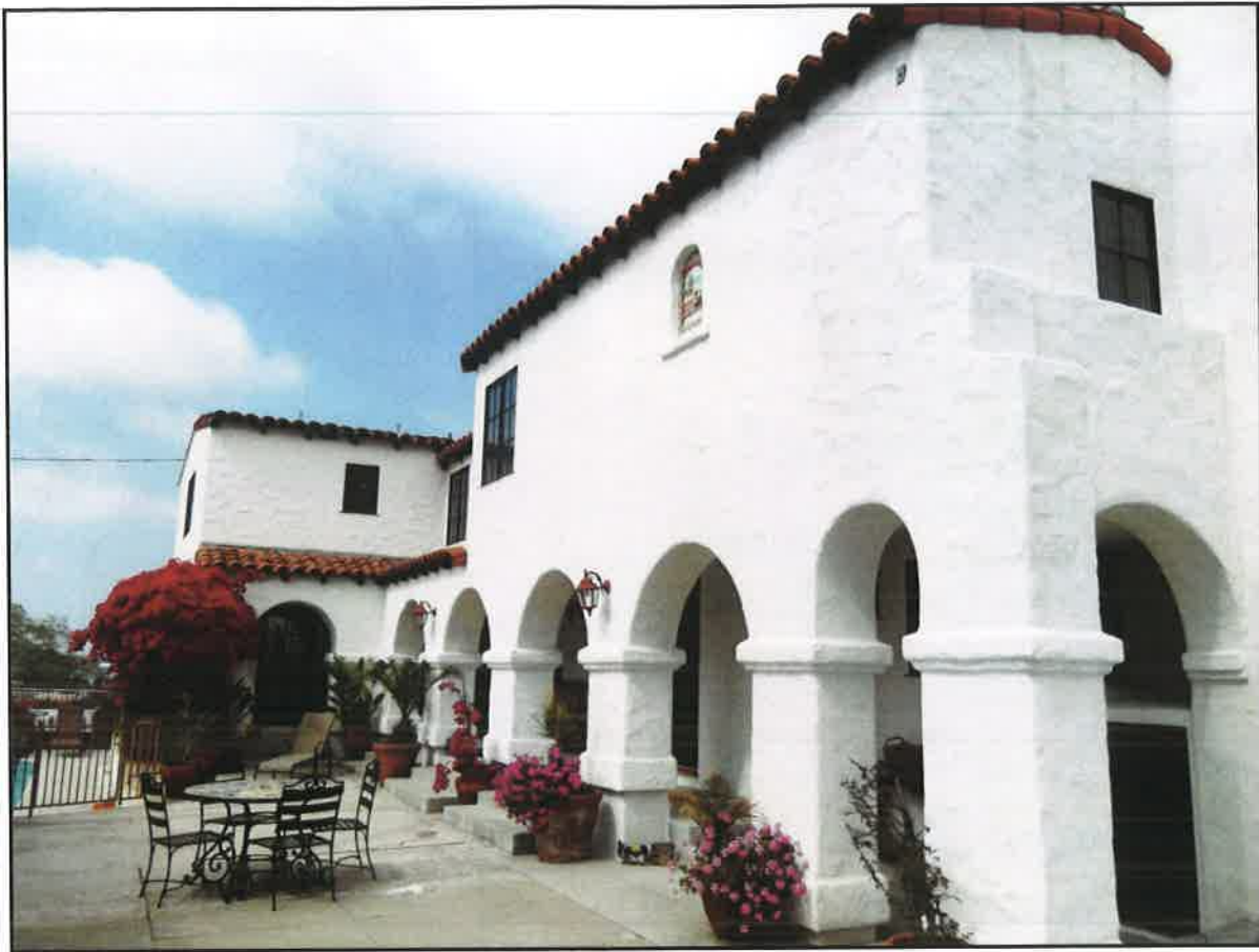
Current Photos - West (rear) Elevation
