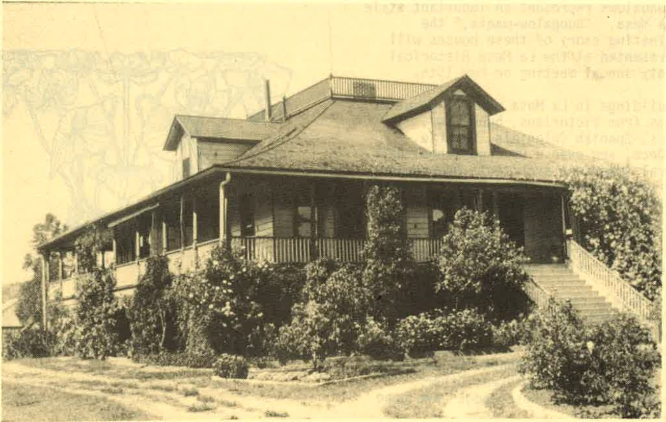
Roach/Porter House c. 1910.
