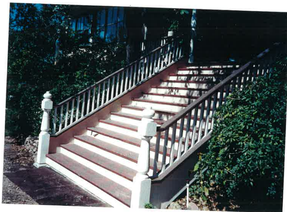
Entrance stairs on the south side.
